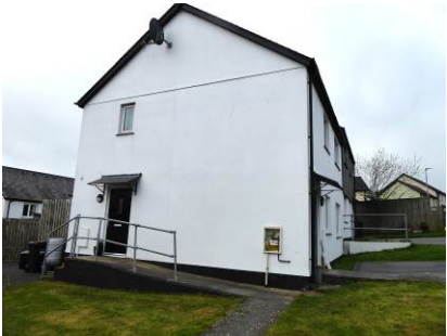
Upper Rowe Court, Dobwalls, Liskeard
