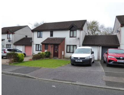
Springfield Close, St Austell
