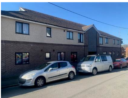
Brookdale Court, Wadebridge
